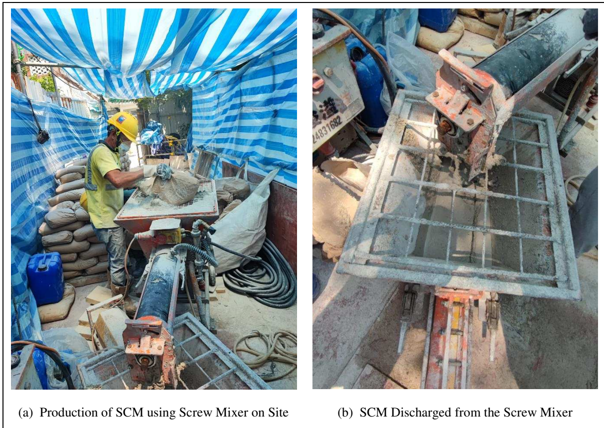
Figure 3.4 Production of Self-compacting Backfill Material Mixed on Site
