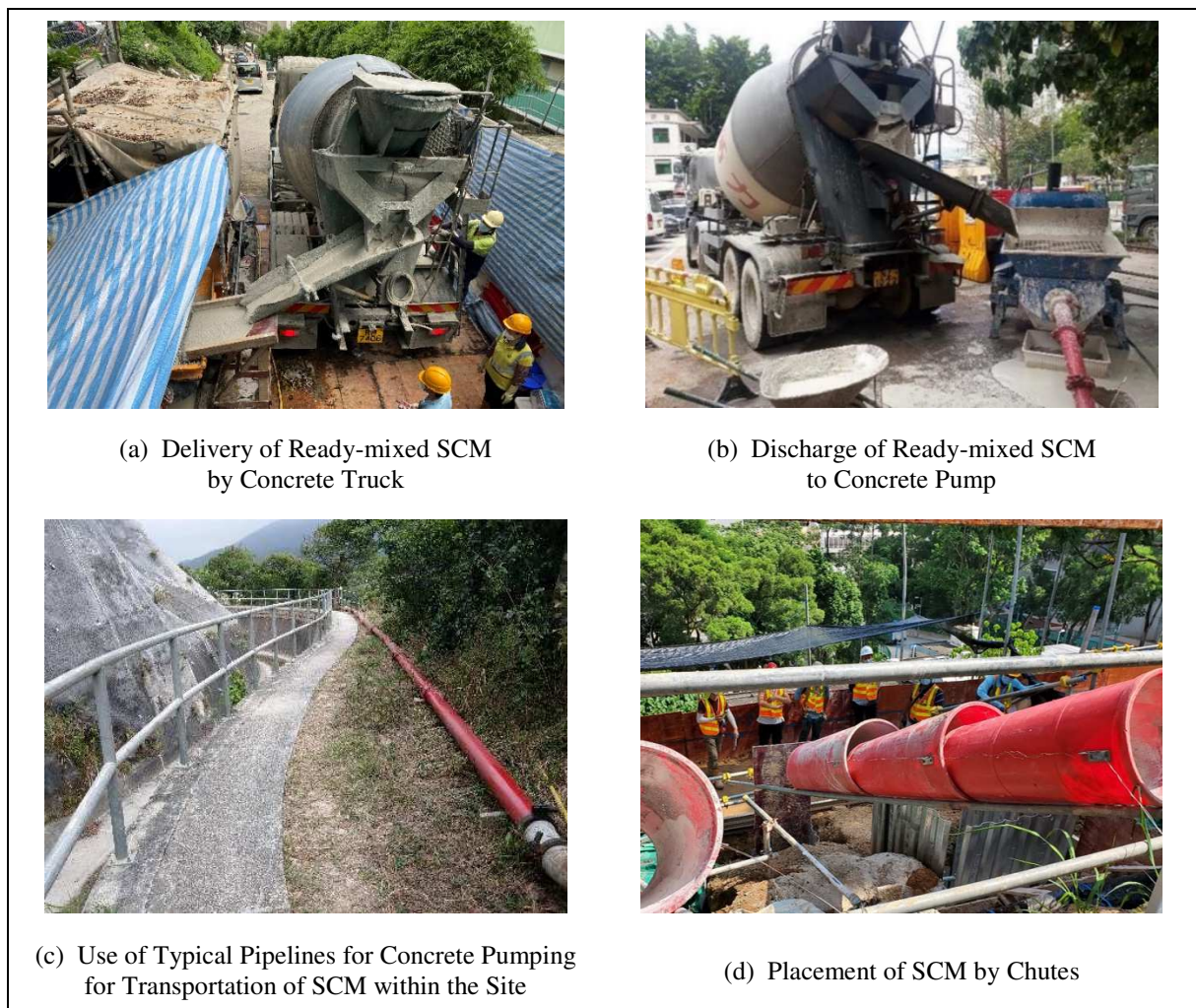
Figure 3.3 Delivery and Placement of Ready-mixed Self-compacting Backfill Material
