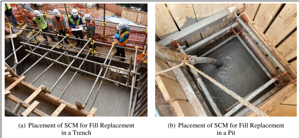
Figure 3.5 Placement of Self-compacting Backfill Material on Site
