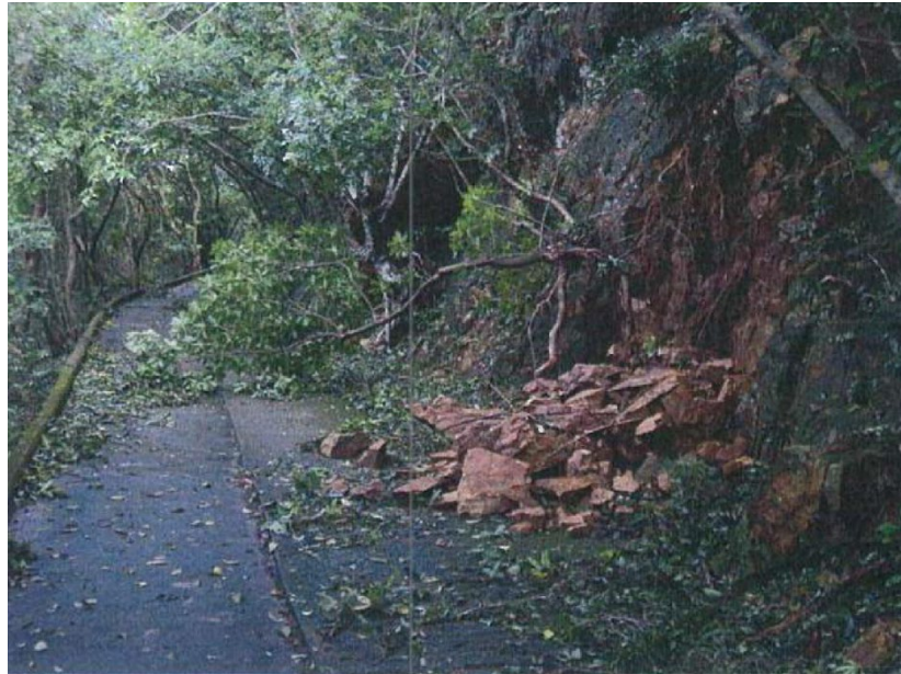
(a) Rockfall on a rock cut slope near Section 4 of Hong Kong Trail, Middle Gap in 2012
