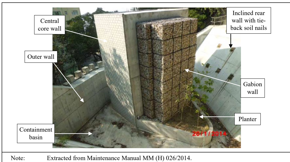
Figure 2.2 Rigid Barrier No. 11SW-C/ND14 (Photograph Taken on 20 January 2014)
