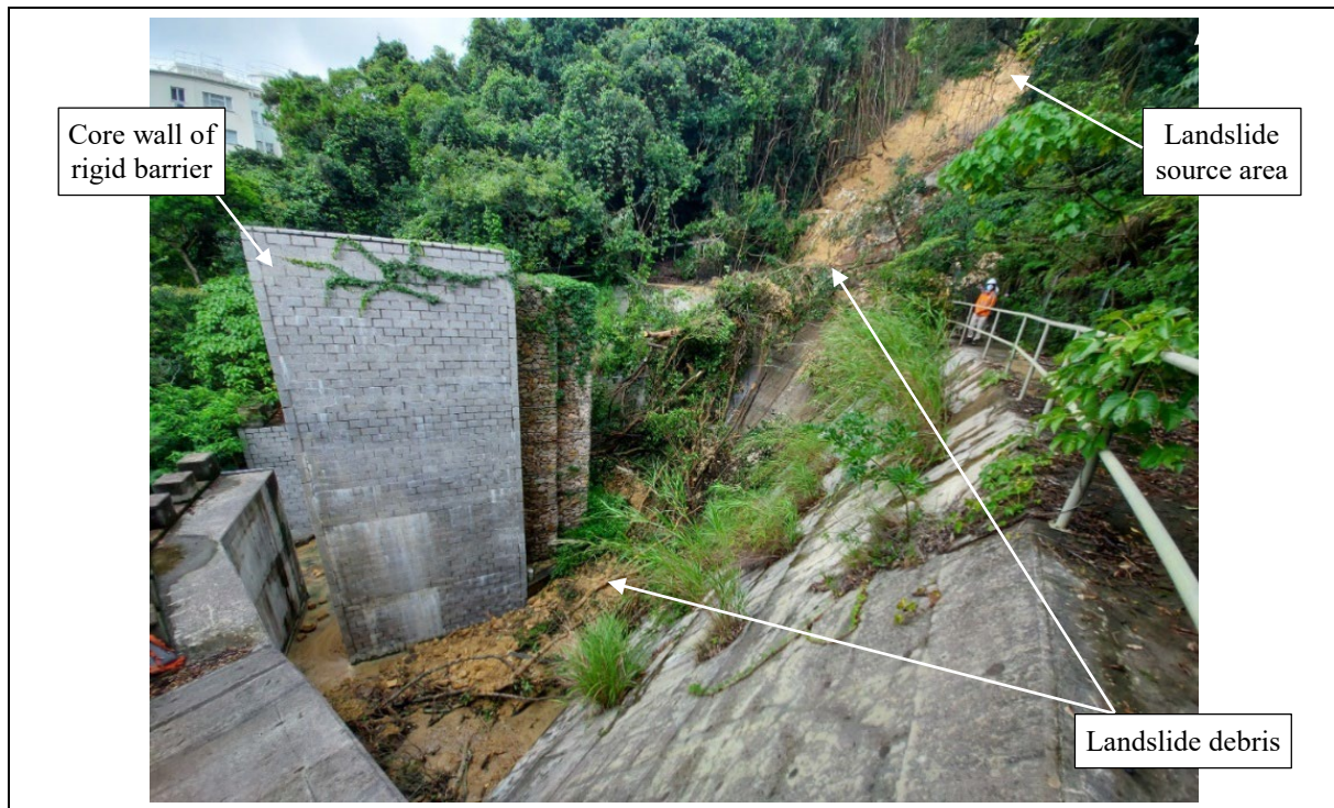
Figure 5.12 View of Landslide Debris Trail (Photograph Taken on 3 August 2021)
