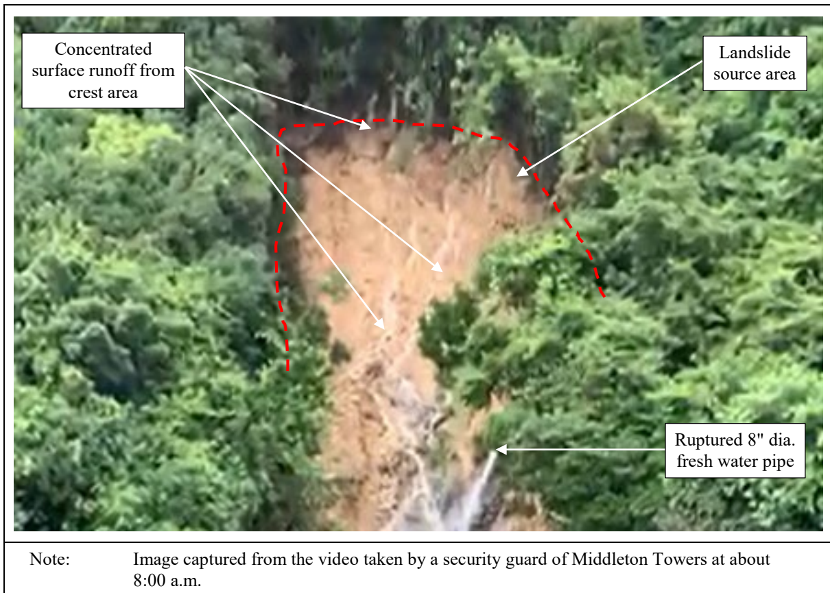
Figure 5.4 Concentrated Surface Runoff from above the Landslide Head Scarp (Video Taken on 3 August 2021)
