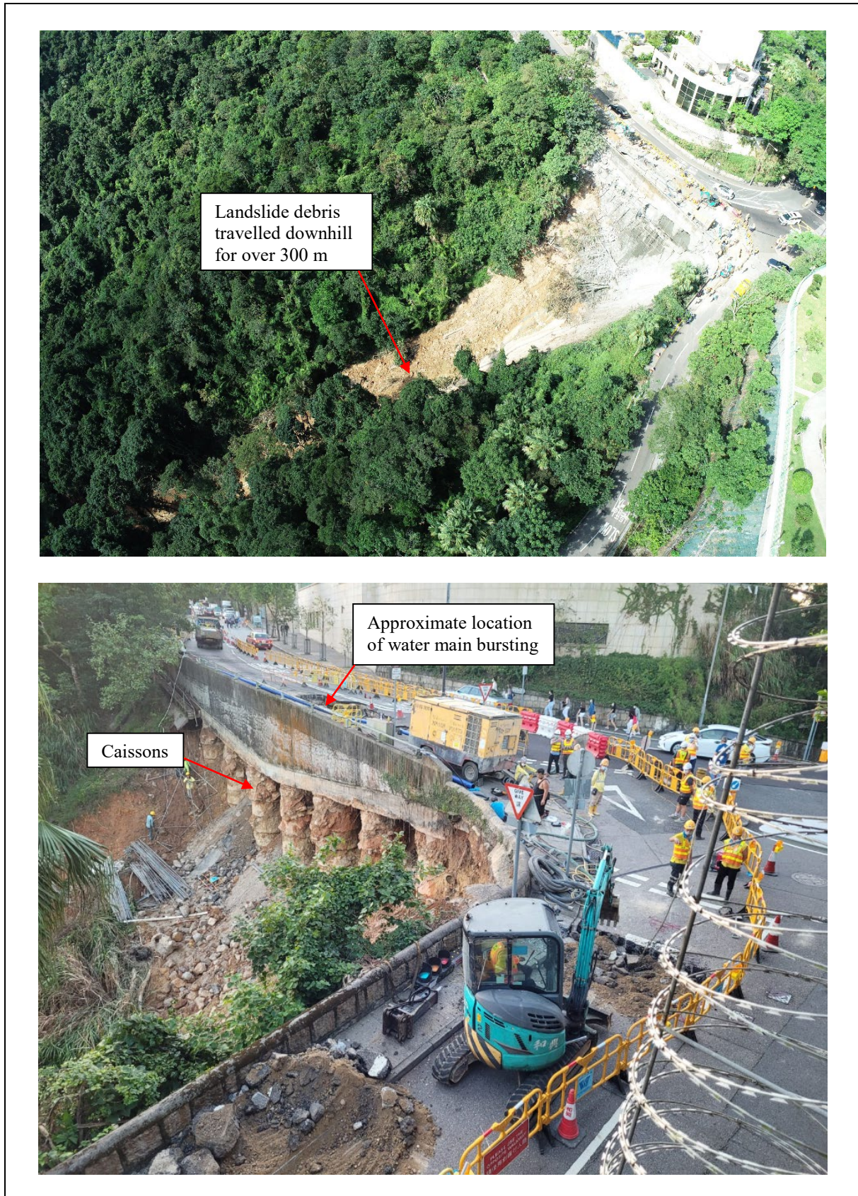
Figure 4.2 Views of the 5 November 2021 Landslide on a Fill Slope at Peak Road, The Peak (Incident No. 2021/11/3089)
