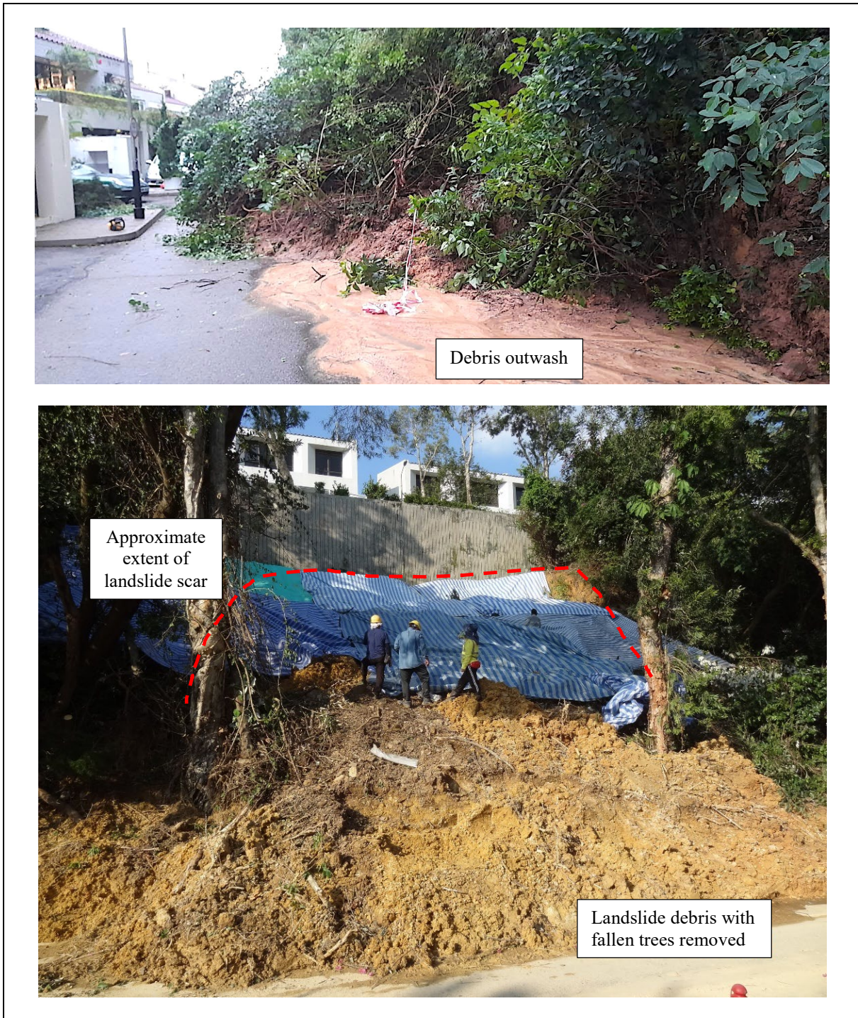
Figure B7 Sliding Failure at Manderly Garden (Incident No. 2021/10/3066)
