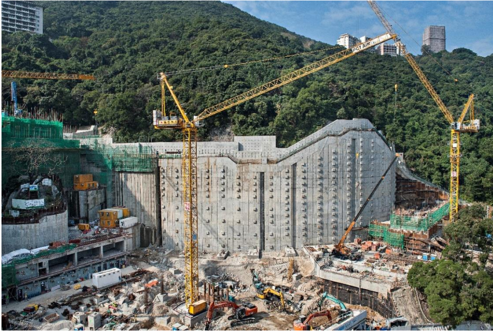
Figure 3.15 Tied-back Wall Support System for the Excavation Works at Stubbs Road
