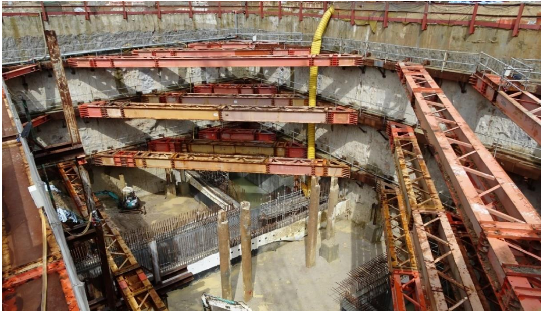
Figure 3.13 Bottom-up Construction
