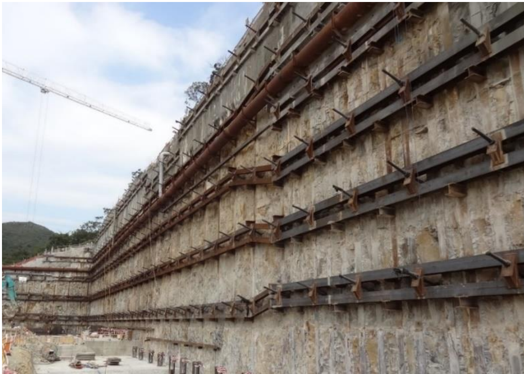
Figure 3.17 Retractable Prestressed Ground Anchor Support System at the Redevelopment of Grantham Hospital
