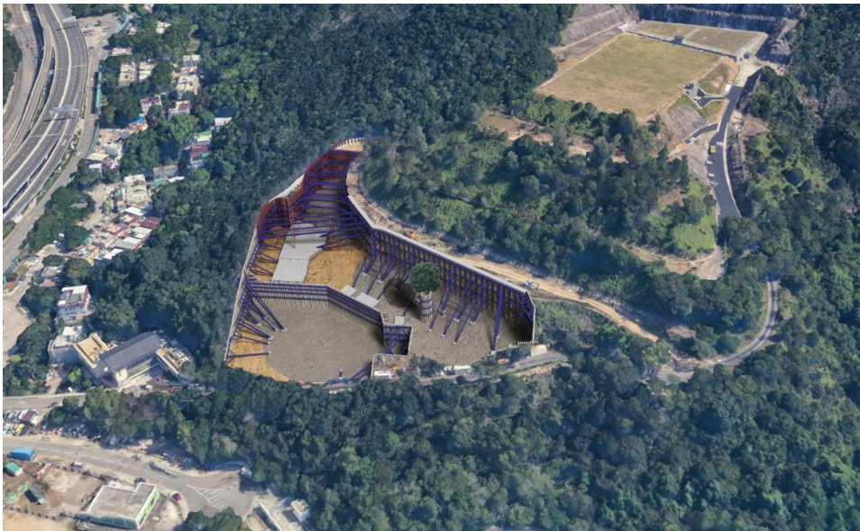
Figure 4.2 Use of BIM for Excavation Works at a Residential Development
