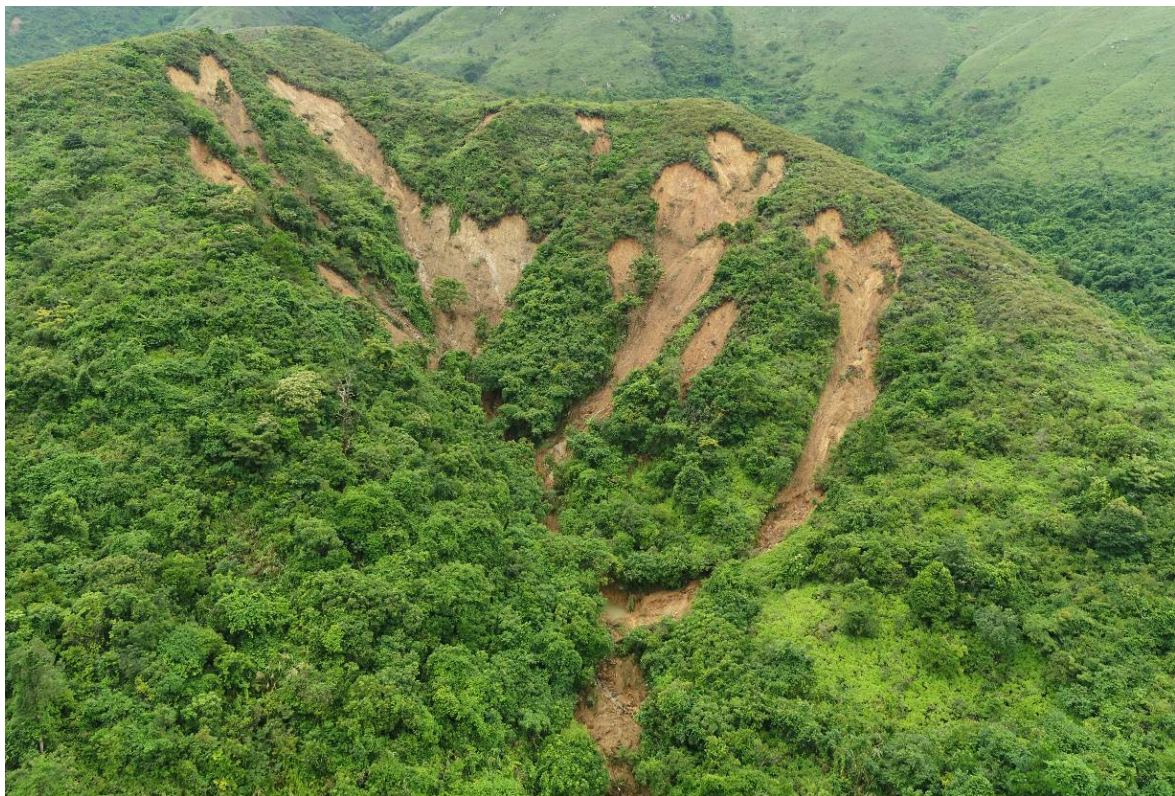
(a) General View of Source Areas of Landslide Cluster 2229
