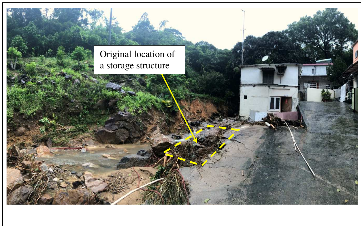
Figure 3.5 A Storage Structure Adjoining to Debris Trail of Landslide Cluster 2228 Reported to have been Washed Away (Photograph taken on 30 August 2018)
