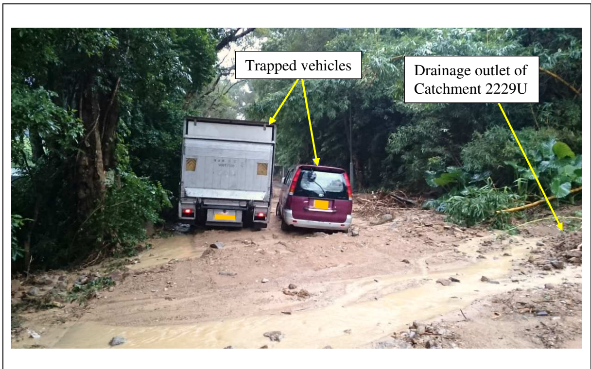
Figure 3.3 View of Outwash Debris on Fan Kam Road from Landslide Cluster 2229U (Photograph taken on 30 August 2018)
