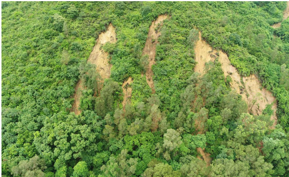
(a) General View of Source Areas of Landslide Cluster 2229L
