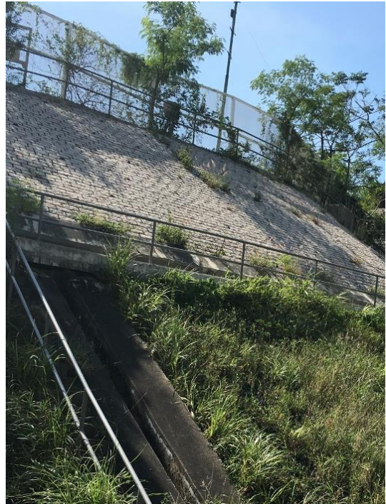
(b) Channel along Interface of Batters below Impermeable Surface Cover
