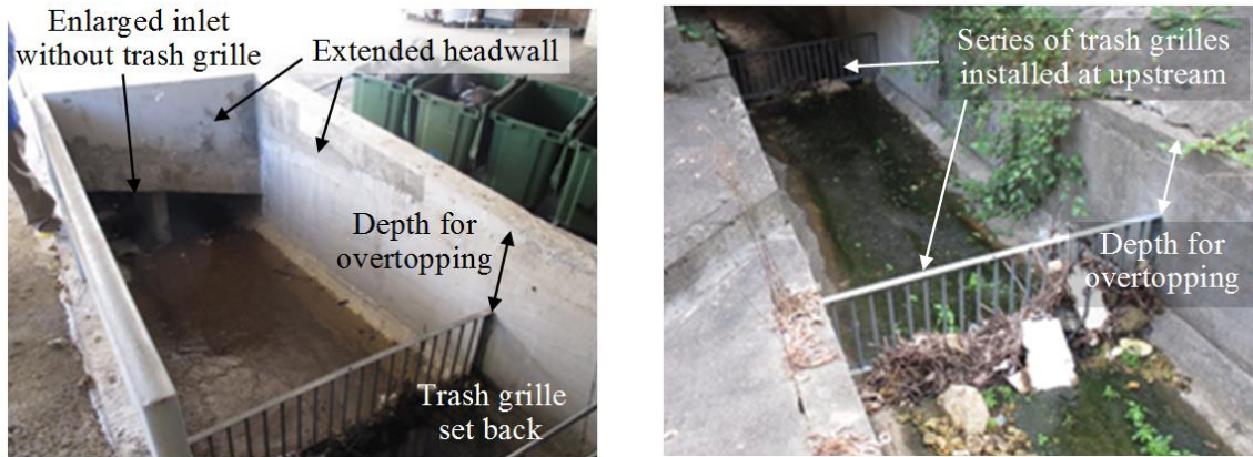
Post-incident Drainage Improvement Measures
