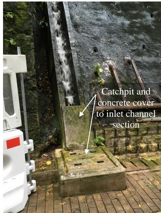
(r) Flow Containment Measure at Connection between Road and Slope Drainage
