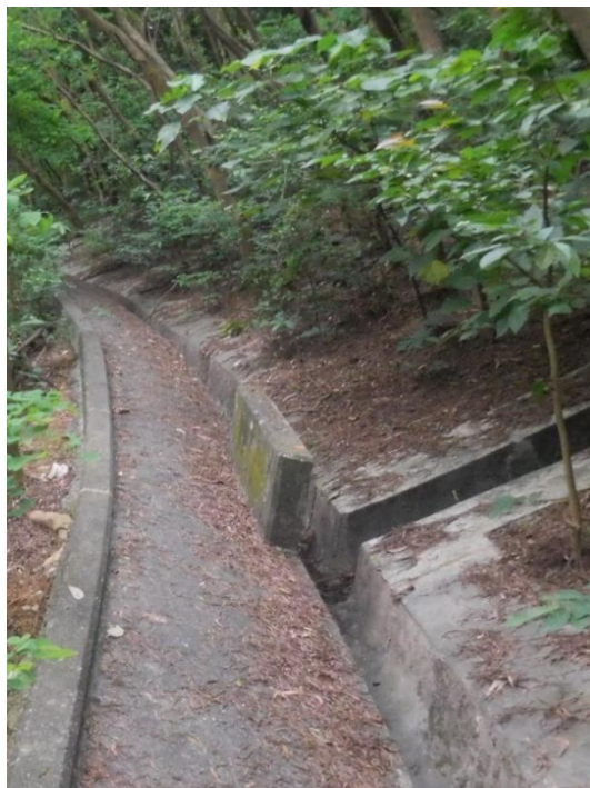
(g) Baffle Wall at Channel Junction as Additional Freeboard
