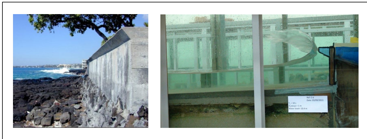
Figure 3.1 Example of a Seawall Recurve and the Associated Laboratory-scale Experiment (Schoonees, 2014)
