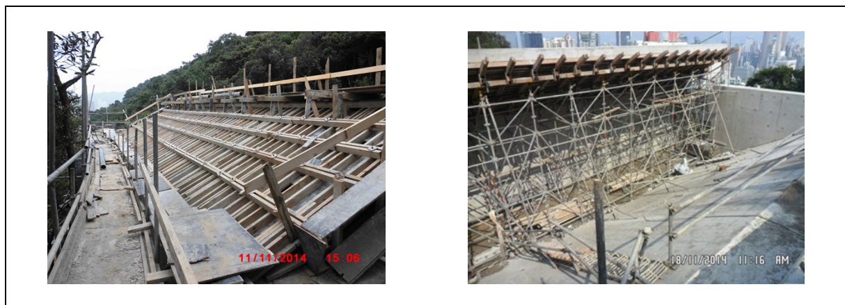
Figure 2.2 Photographs Showing the Construction of a Deflector
