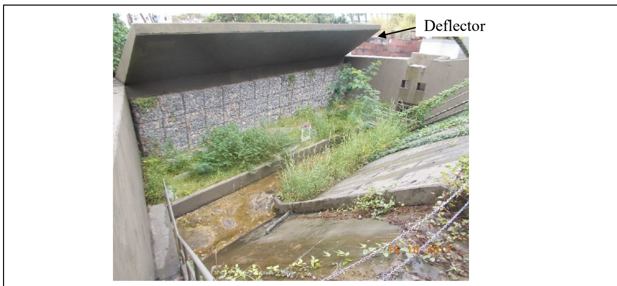
Figure 1.1 Example of a Deflector Constructed in Bowen Road
