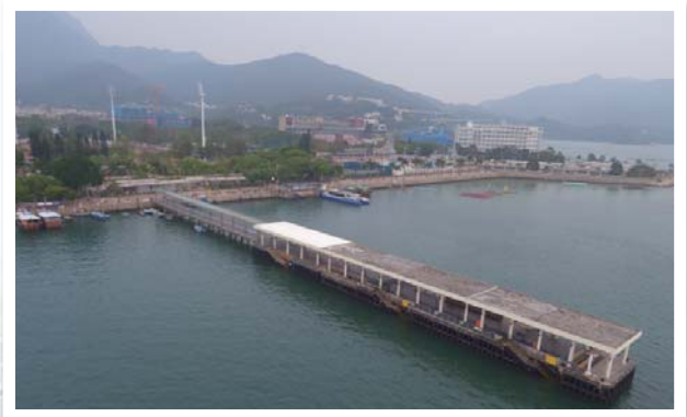
Improvement works to Sai Kung Public Pier
