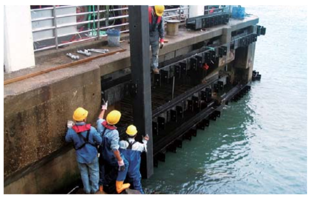
Fender upgrading works at the pier
