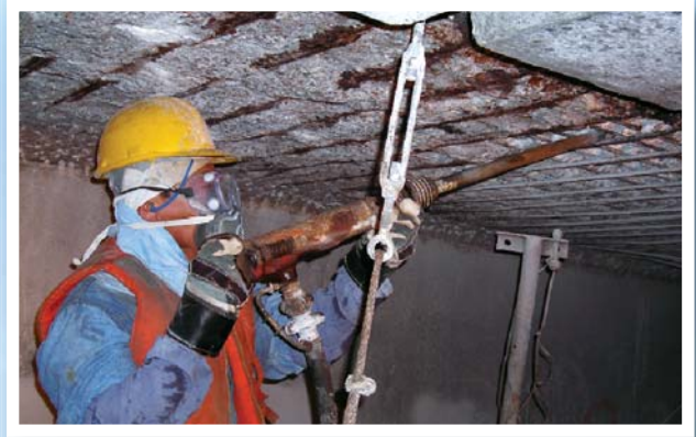
Concrete repair works at the pier
