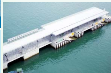
Sai Kung New Public Pier
