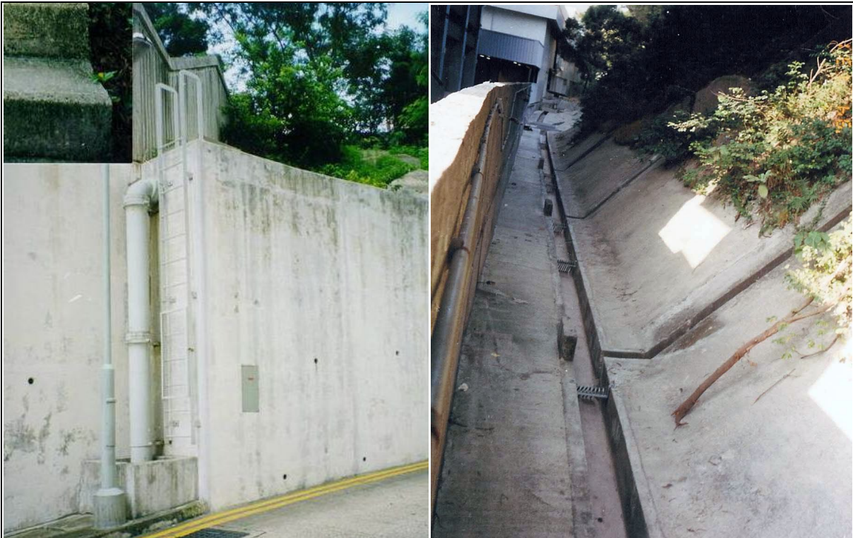
(a) Exposed Down Pipe on Retaining Wall
