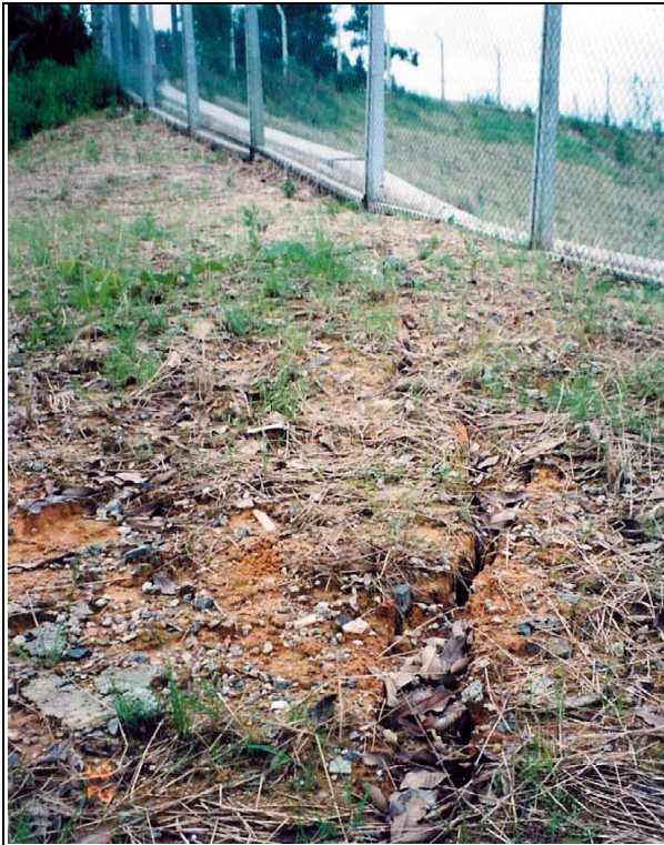
(a) Tension Crack on Slope
