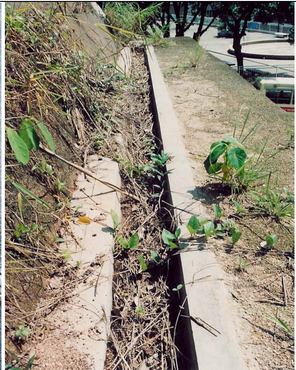
(b) U-channel along Berm of Slope
