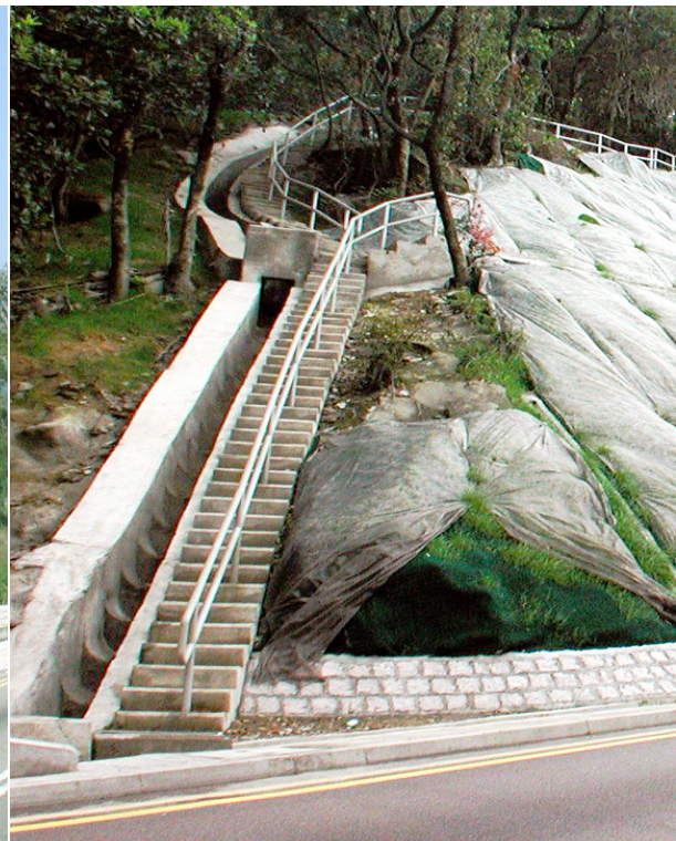
(d) Combined Stepped Channel and Stairway
