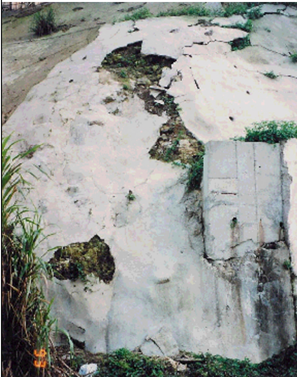
(c) Cracked Chunam Surface
