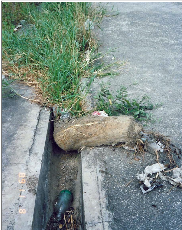
(a) U-channel along Crest of Slope
