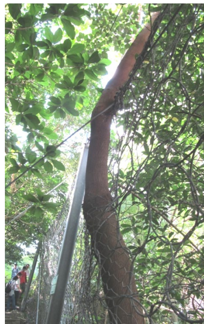
Tree passing through principal net of barrier
