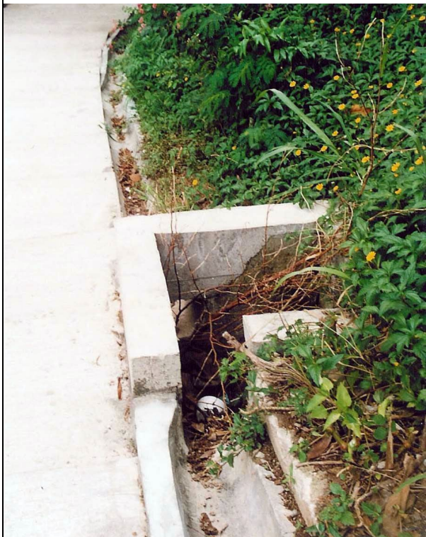
(c) Catchpit at Toe of Slope
